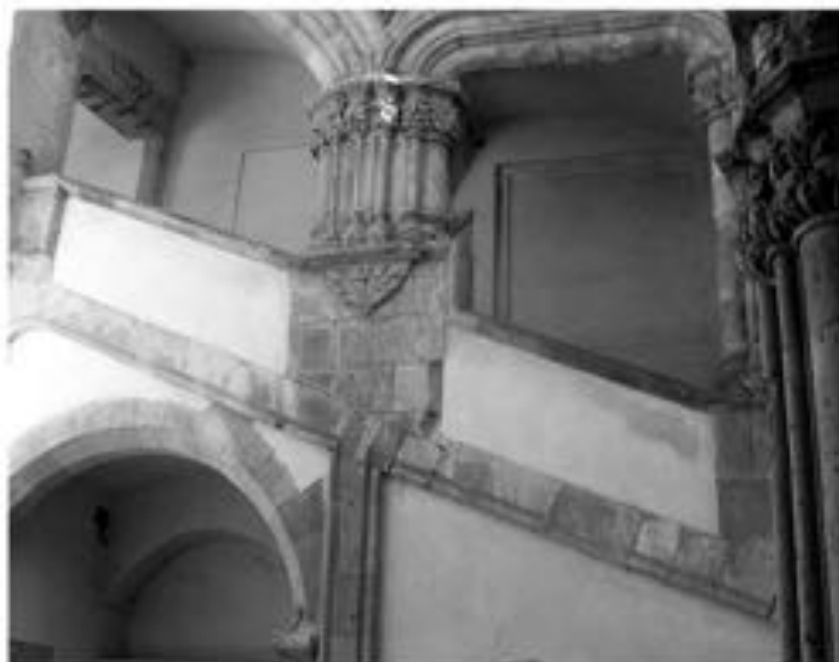
Fig. 1 - Carinola (CE), Palazzo Marzano, view of the court yard (XV century)
